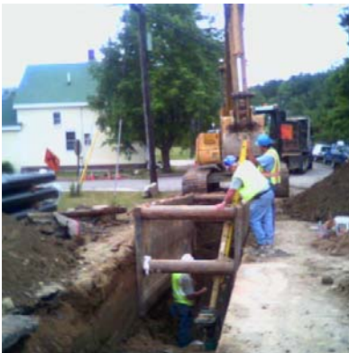
Contractors install water main on Churchill Street during a 2008 District project
