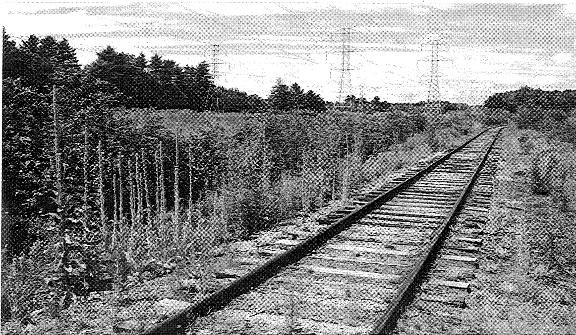
The rail spur north of Route 144.
