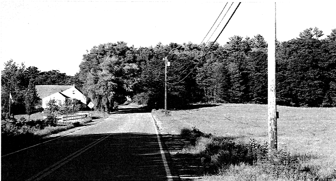
Route 144 at the north end of the Ferry Road North site, on right of photo.
